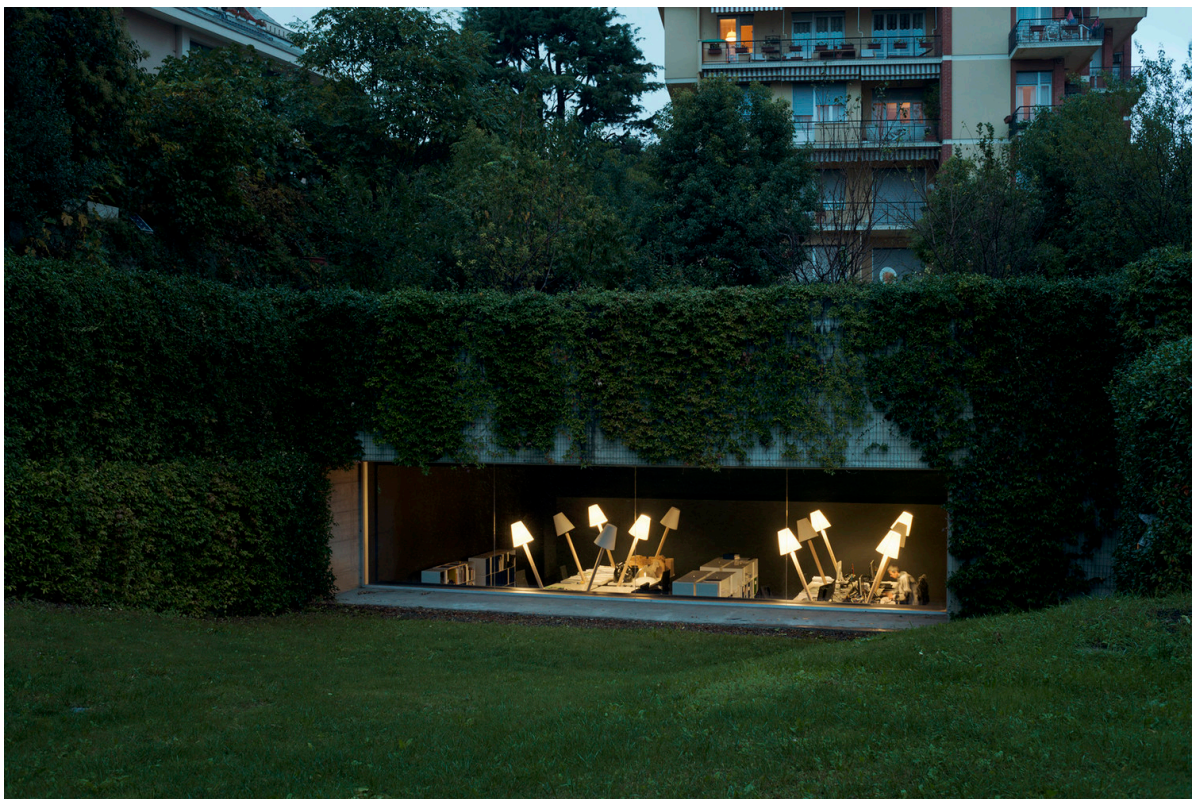
Bild 15: Underground Garage Genua, von Carlo Bagliani, https://www.archdaily.com/460641/underground-garage-carlo-bagliani
